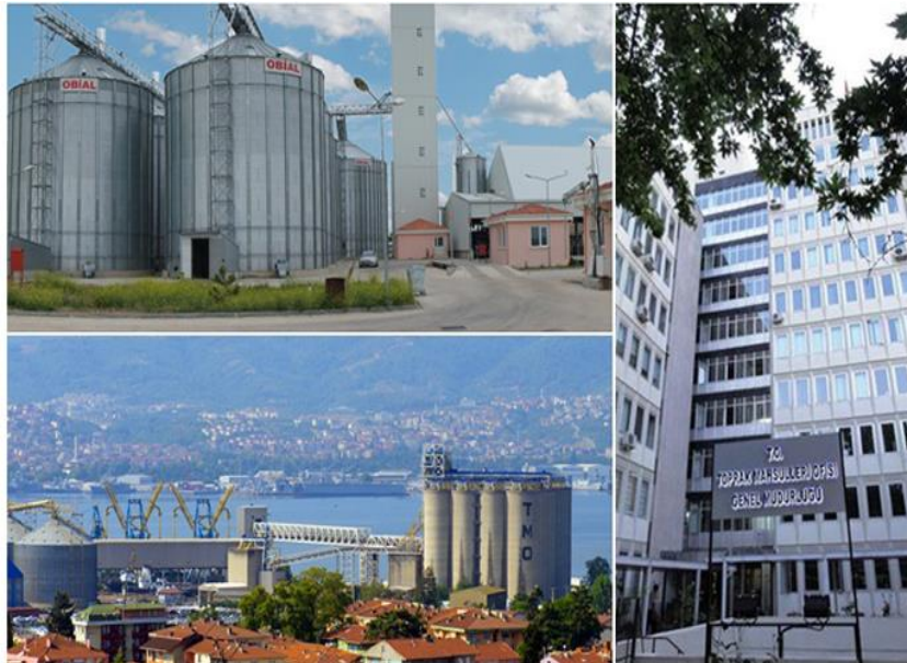
TMO's headquarter building in Ankara and its various silos
